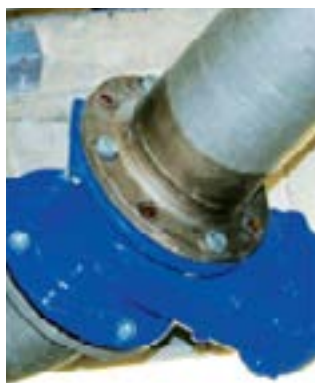
REPLACEMENT OF A GATE VALVE WITH BUTTERFLY VALVE WITH LOOSE FLANGE.
