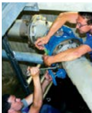
REPLACEMENT OF A GATE VALVE WITH BUTTERFLY VALVE WITH LOOSE FLANGE.
